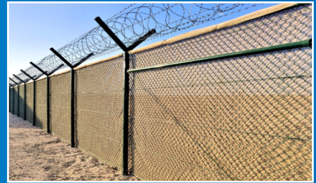
Barbed wire Fencing
